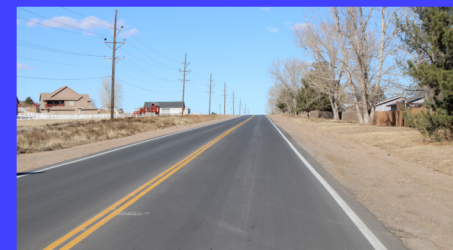
47th Avenue asphalt reconstruction
