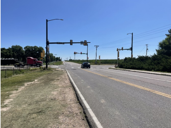
NW corner of Intersection - Facing West (August 2023)
