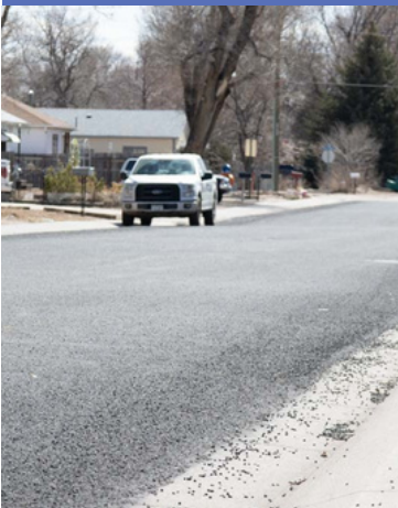
Chip seal work completed in 2022 in East Evans
