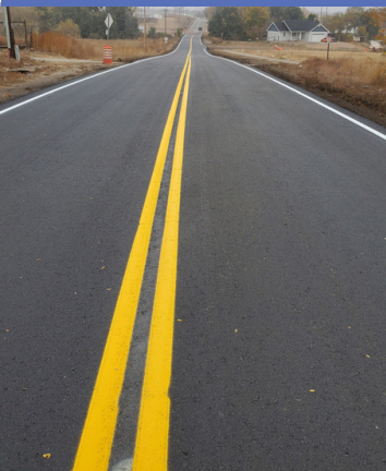
Mill and overlay work on 49 th St. in 2023
