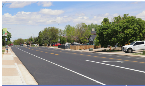
Completed mill & overlay work on 17 th Ave.
